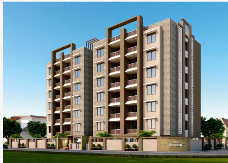
VIMAL APARTMENT - COMPLETED
