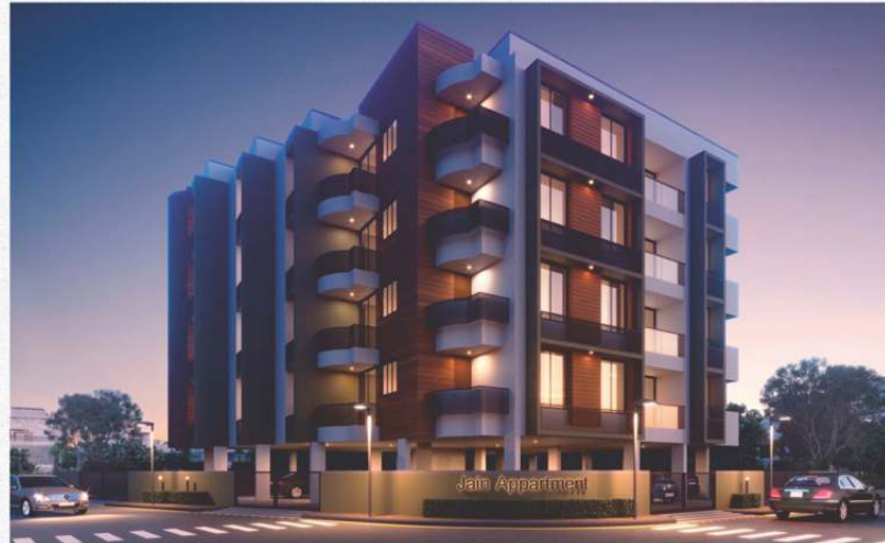
JAIN APARTMENT - COMPLETED
