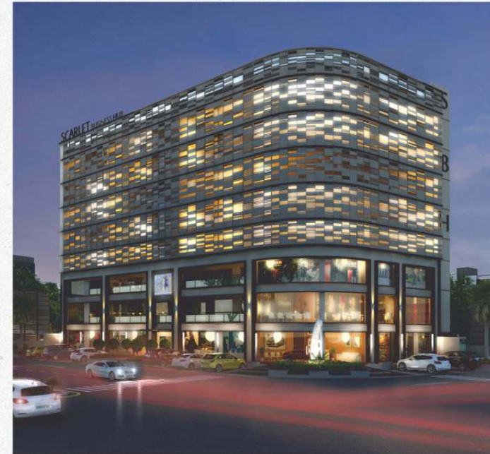
SCARLET BUSINESS HUB - COMPLETED
