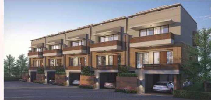
ON GOING PROJECT SAMARTHYA HOMES @ 2018
