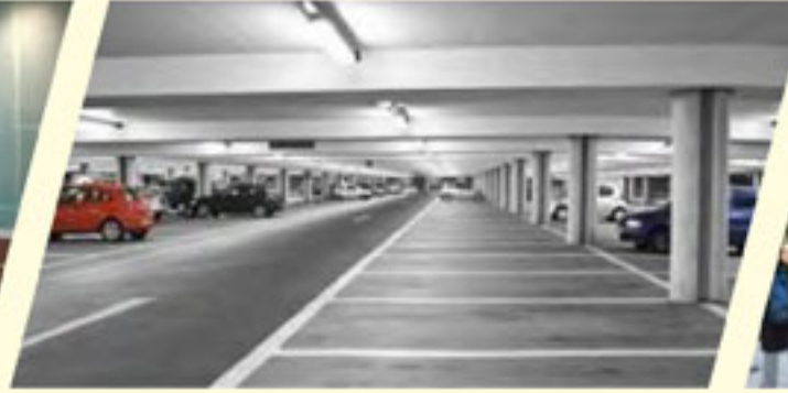
Podium parking with internal driveways
